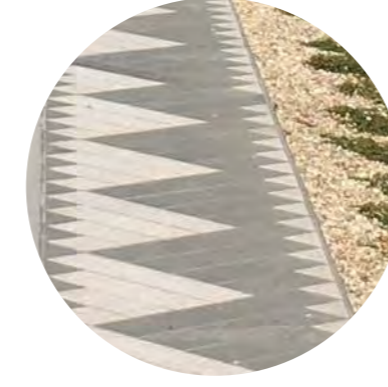
STONE PAVING STRIP 40mm stone paving cut and laid to pattern
