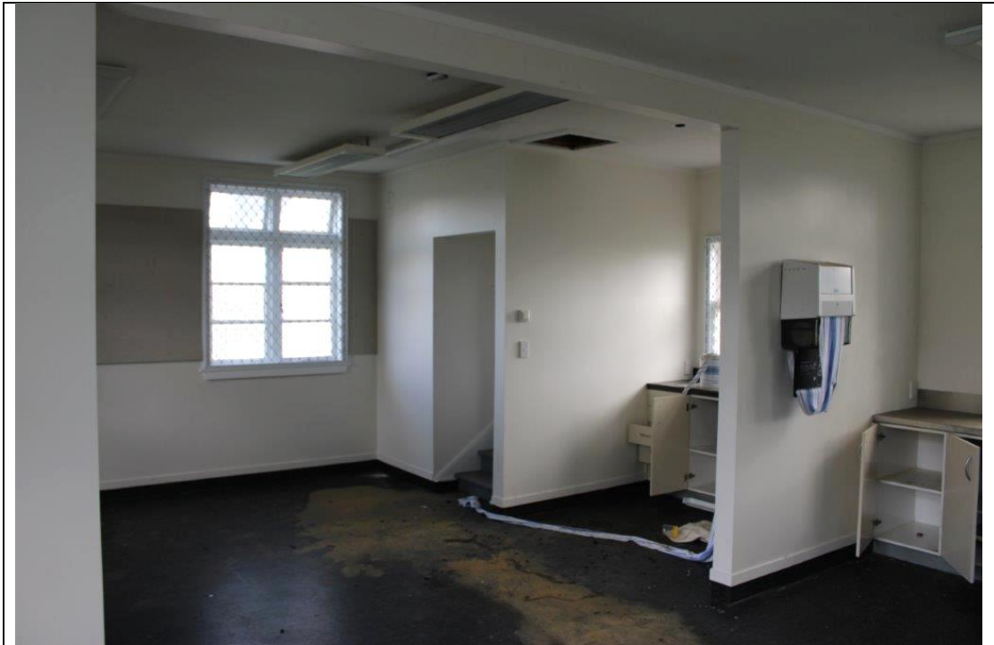
The western end of the building. Kitchen cabinetry is a later modification.
