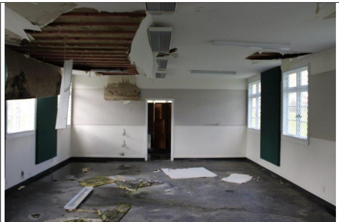
Inside the main classroom space looking towards the room located at the eastern end of the building.
