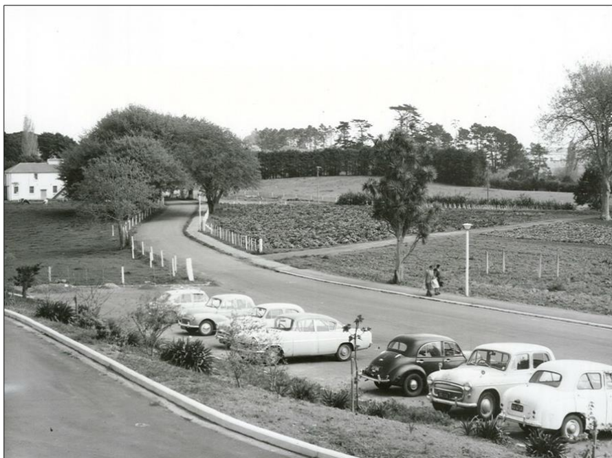
Figure 9 Oakley Hospital market gardens in 1967 with Building 28 at left rear. The exterior staircase appears in tact. R24730973, Archives New Zealand Auckland repository, photographer Gerald Riethmaier.
