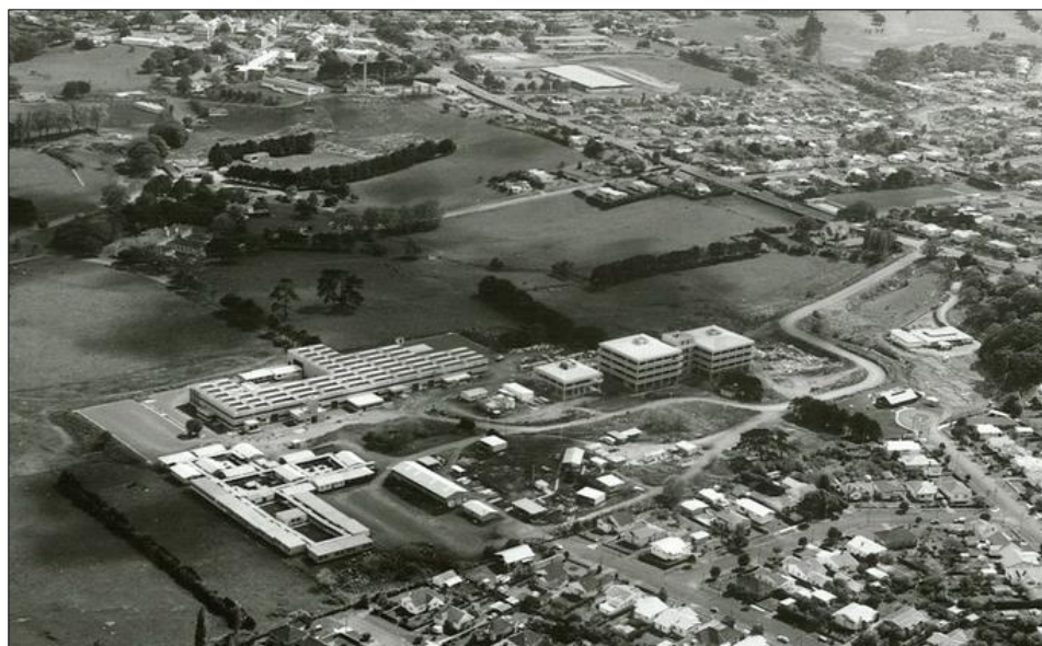
Figure 18: Buildings of Carrington Technical Institute in 1977. R24815830, Archives NZ.
