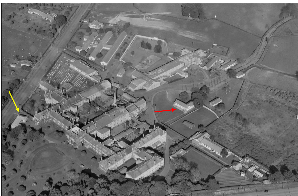
Figure 6 A 1949 photograph showing Building 203 indicated with red arrow and the New Zealand Occupational Therapy Training School indicated with yellow arrow. Alexander Turnbull Library WA-20753-F.
