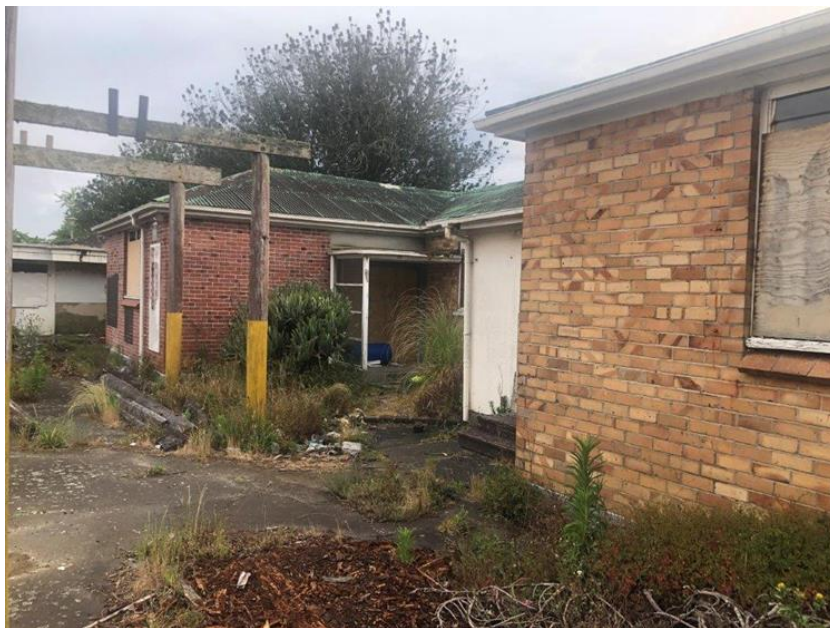
Figure 4 Present-day views of the former New Zealand Occupational Therapy Training School building built in 1946 (honey coloured brick building at right) and extended in 1954 (at left) adjacent to Carrington Road at the northeast end of the former hospital site. DPA Architects .
