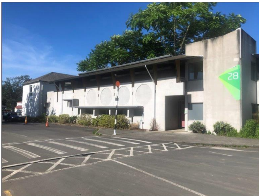
Figure 12 Photographs of the heritage building incorporated into the Unitec Landscape and Plant Sciences building designed by Mitchell Stout Architects connected to it. DPA Architects.
