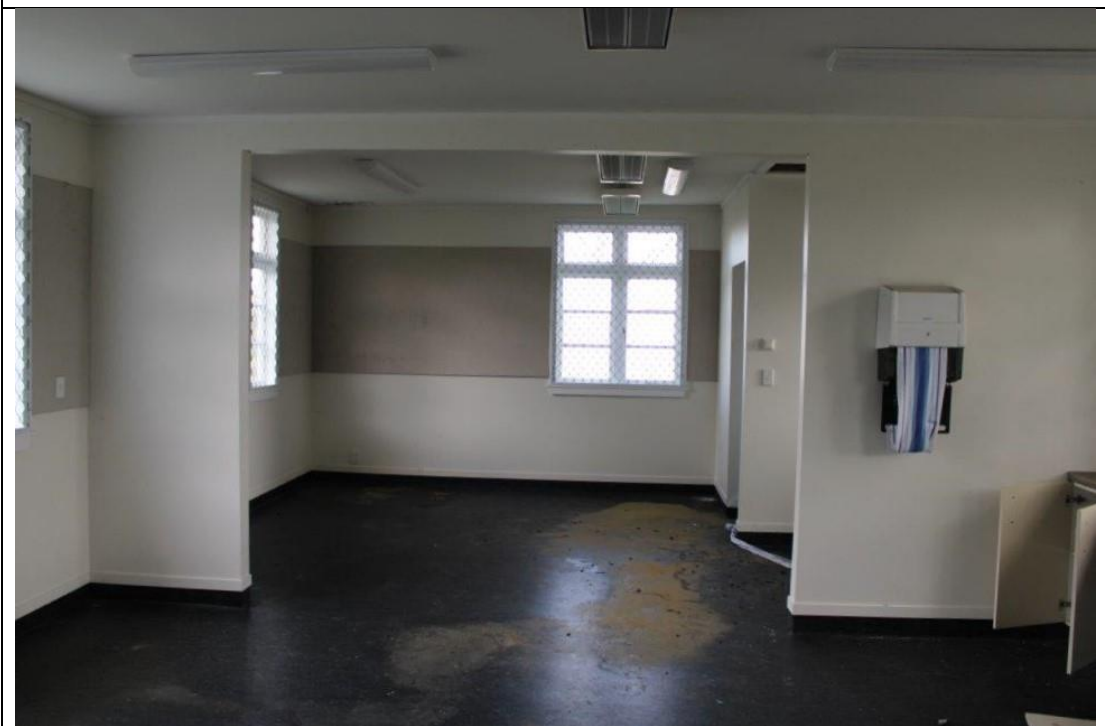
Looking west from the entrance space. The opening within this wall is not believed to be original.
