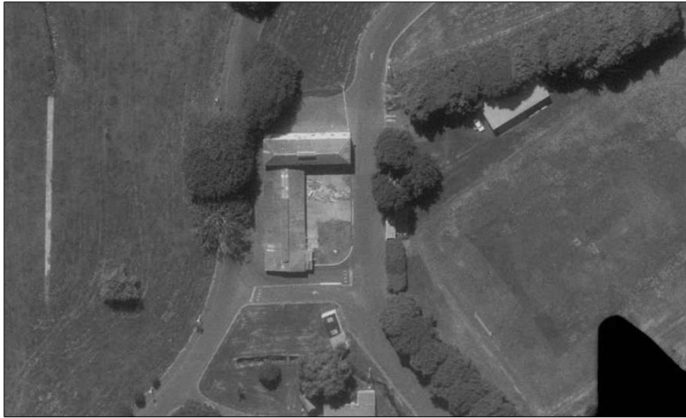
Figure 10 A 1985 aerial photograph shows the milking sheds complex only partially intact, with Building 28 and the single level building at right angles to it remaining. Survey number SN8515, 28 March 1985, retrolens.co.nz .
