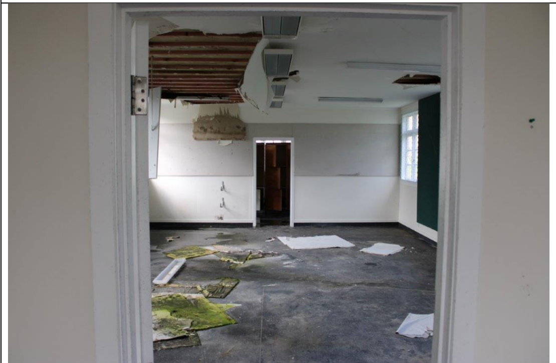
Looking east from the entrance into the main classroom space. A smaller room is located beyond this space, at the east end of the building.
