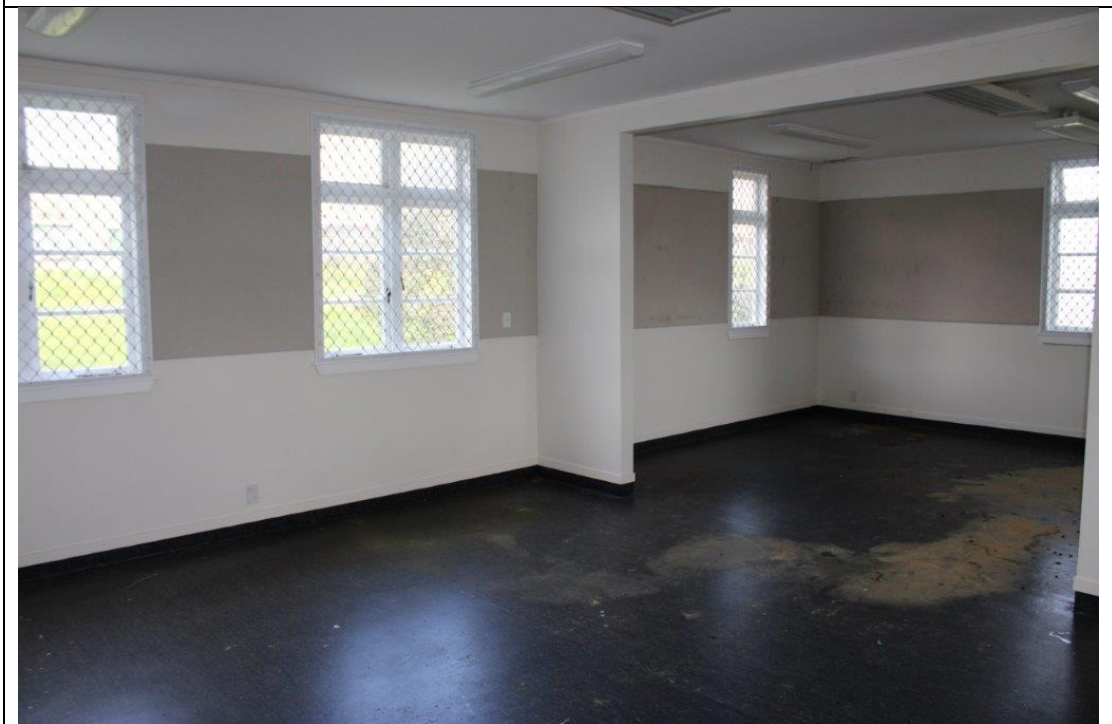
The southwestern end of the building. Walls and ceilings appear to have been relined with plasterboard. The floor is vinyl.
