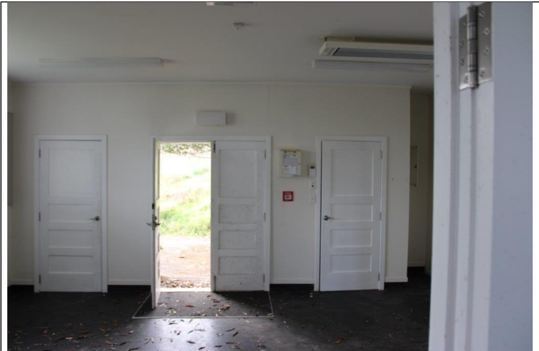
Inside the entrance, looking north. Timber panelled cupboard doors are located either side of the timber panelled double entrance doors.
