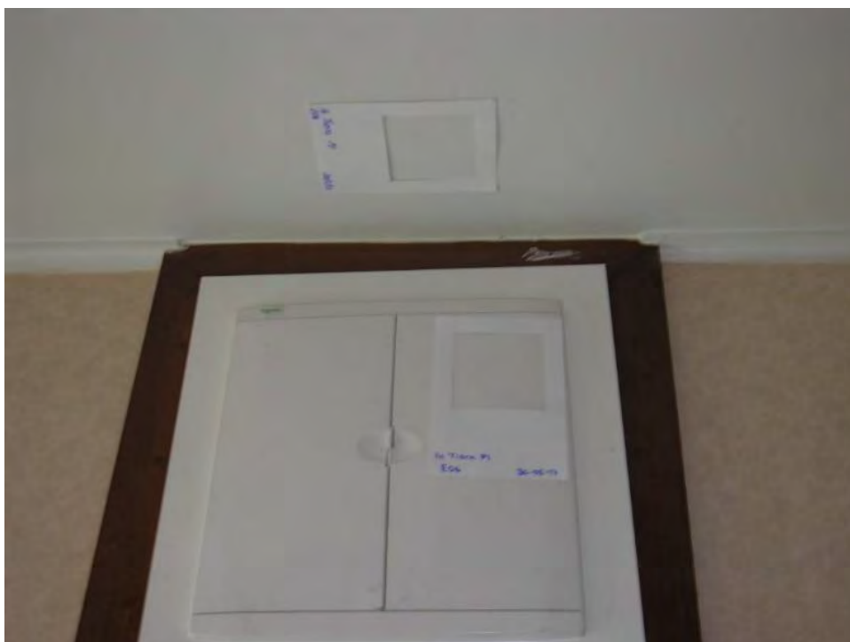
Photograph 15: Sampling sites in the centre of the ceiling in the entry hallway and the fuse box cover.
