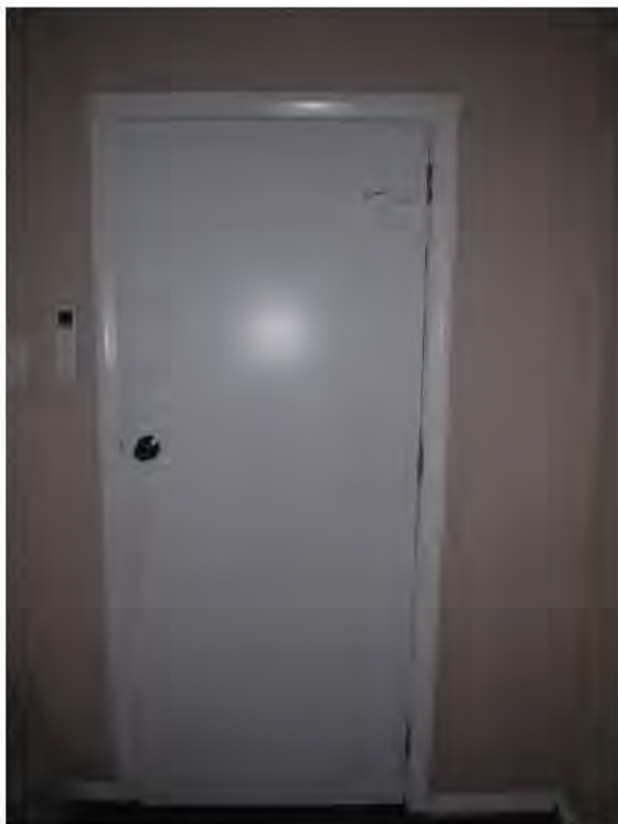
Photograph 3: Sampling sites on the door in the lounge.
