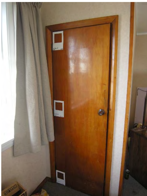
Photograph 11: Sampling sites on the varnished door in bedroom 1.
