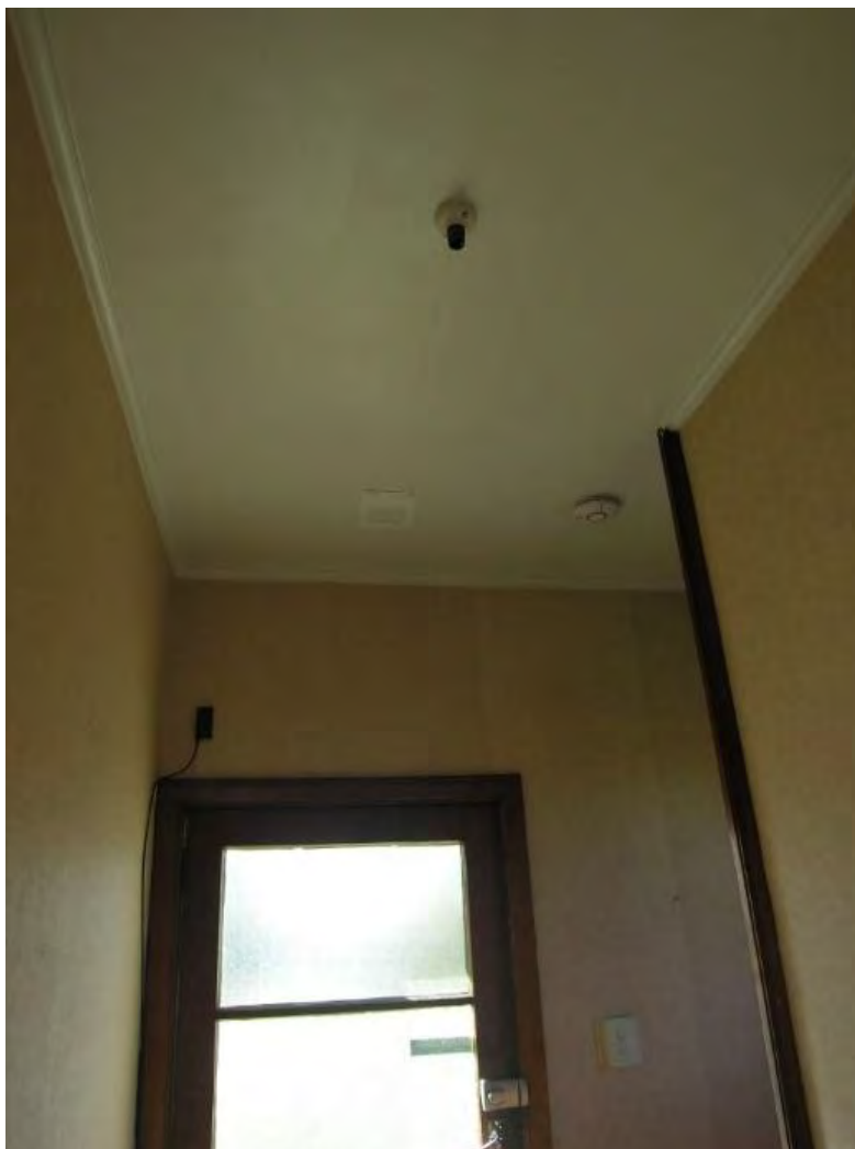
Photograph 14: Sampling site on the ceiling in the entry hallway close to the front door.
